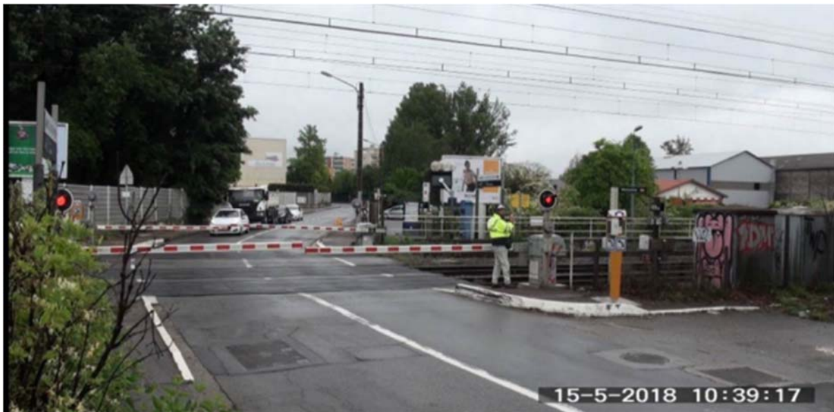
Figure 3: A first view of the Montaudran level crossing
