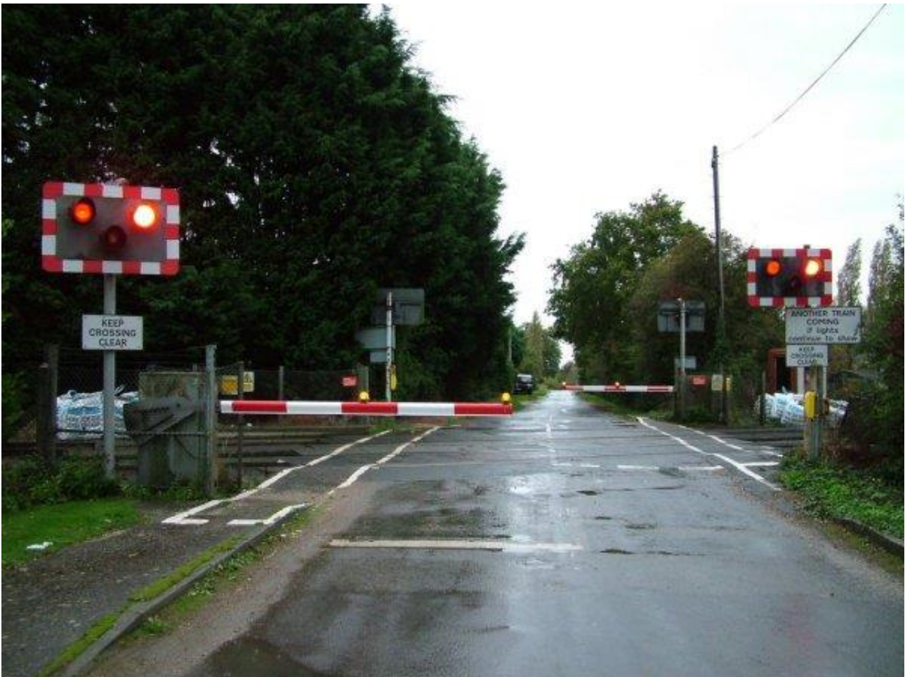
Figure 61. Flashing Lights and Barriers example.
