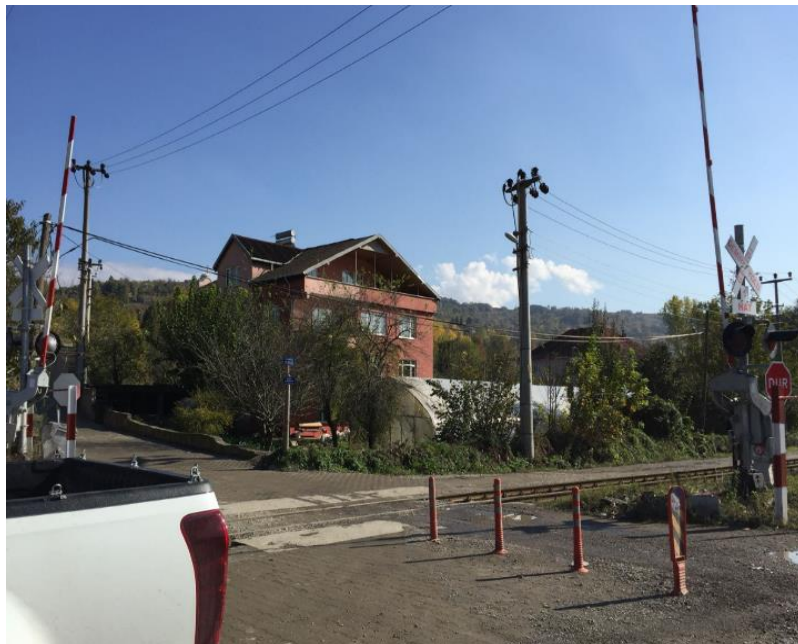
Figure 66. Implementation site 2 Coloured Pavement Markings.
