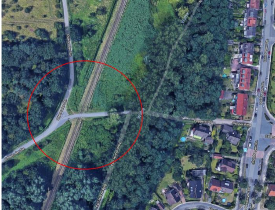
Figure 51. Passive LC at Ottenroder Straße, Braunschweig (aerial view).
