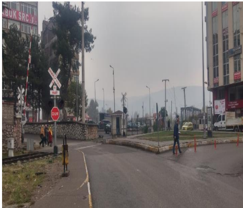
Figure 67. Implementation site 1 Flashing Lights on the Barriers.
