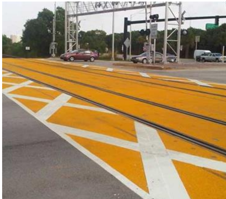
Figure 62. Coloured Pavement Markings example.
