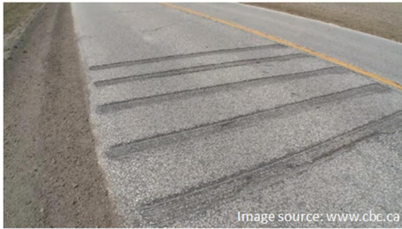
Figure 4. Rumble strips and other purposeful alterations of the road surface are supposed to influence the driving behavior of motorized road users during the approach towards level crossings.
