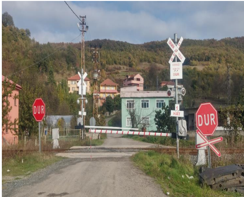
Figure 65. Implementation site 1 Coloured Pavement Markings.
