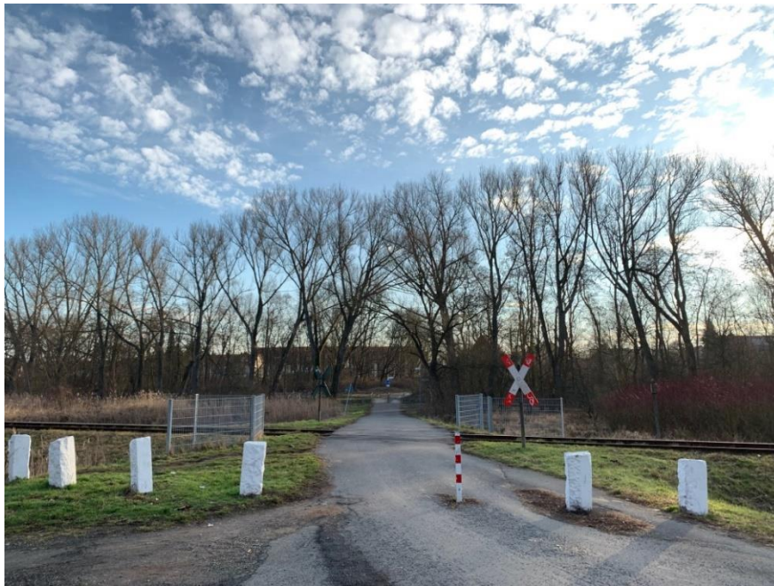
Figure 52. Passive LC at Ottenroder Straße, Braunschweig (western approach view).
