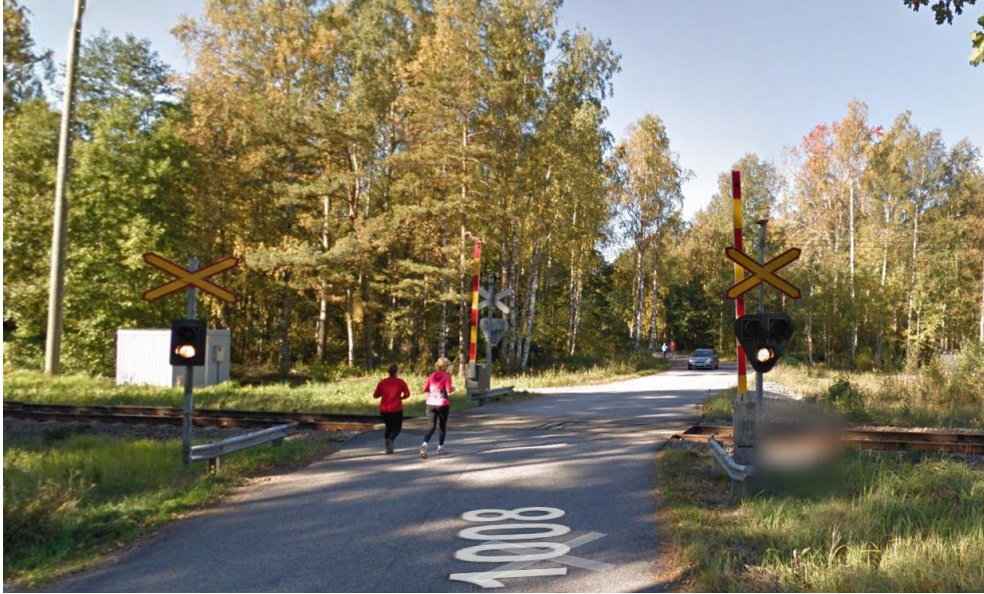
Figure 12. Level crossing Kirkkotie used in simulation © Google Street View.
