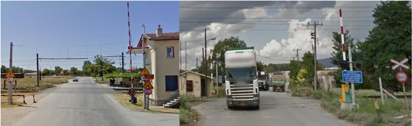
Figure 60. Two of the three level crossings studied, fitted with appropriate road signals, protective barriers, warning alarms and flashing lights. Photos from Google Street View.
