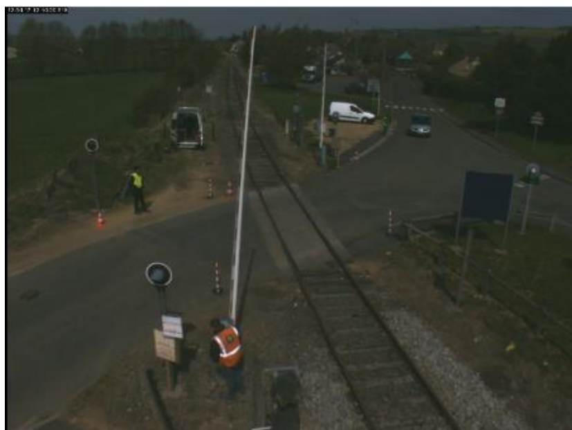
Photo 2: Mouzon test site
