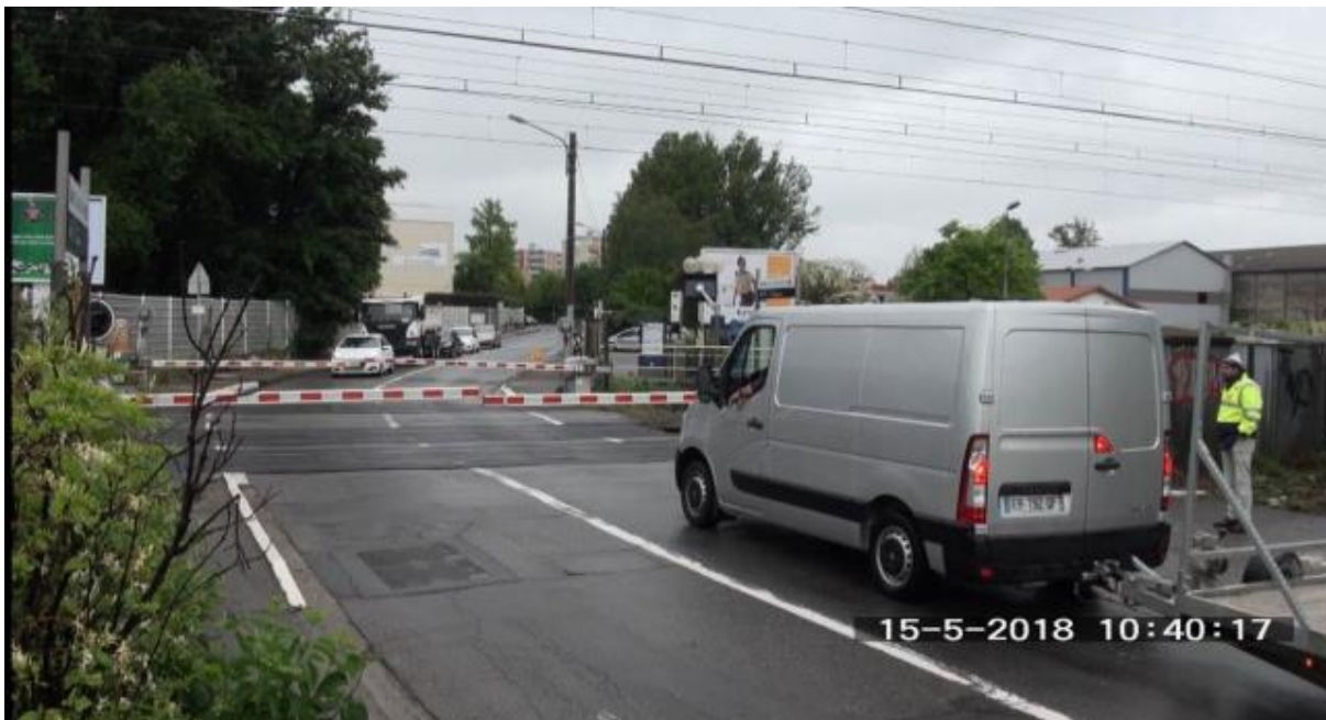
Photo 4: Another picture shot at Montaudran test site
