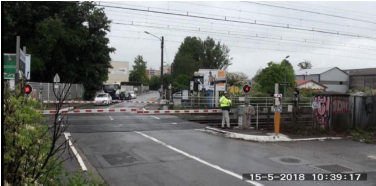
Photo 3: A first view of the Montaudran level crossing
