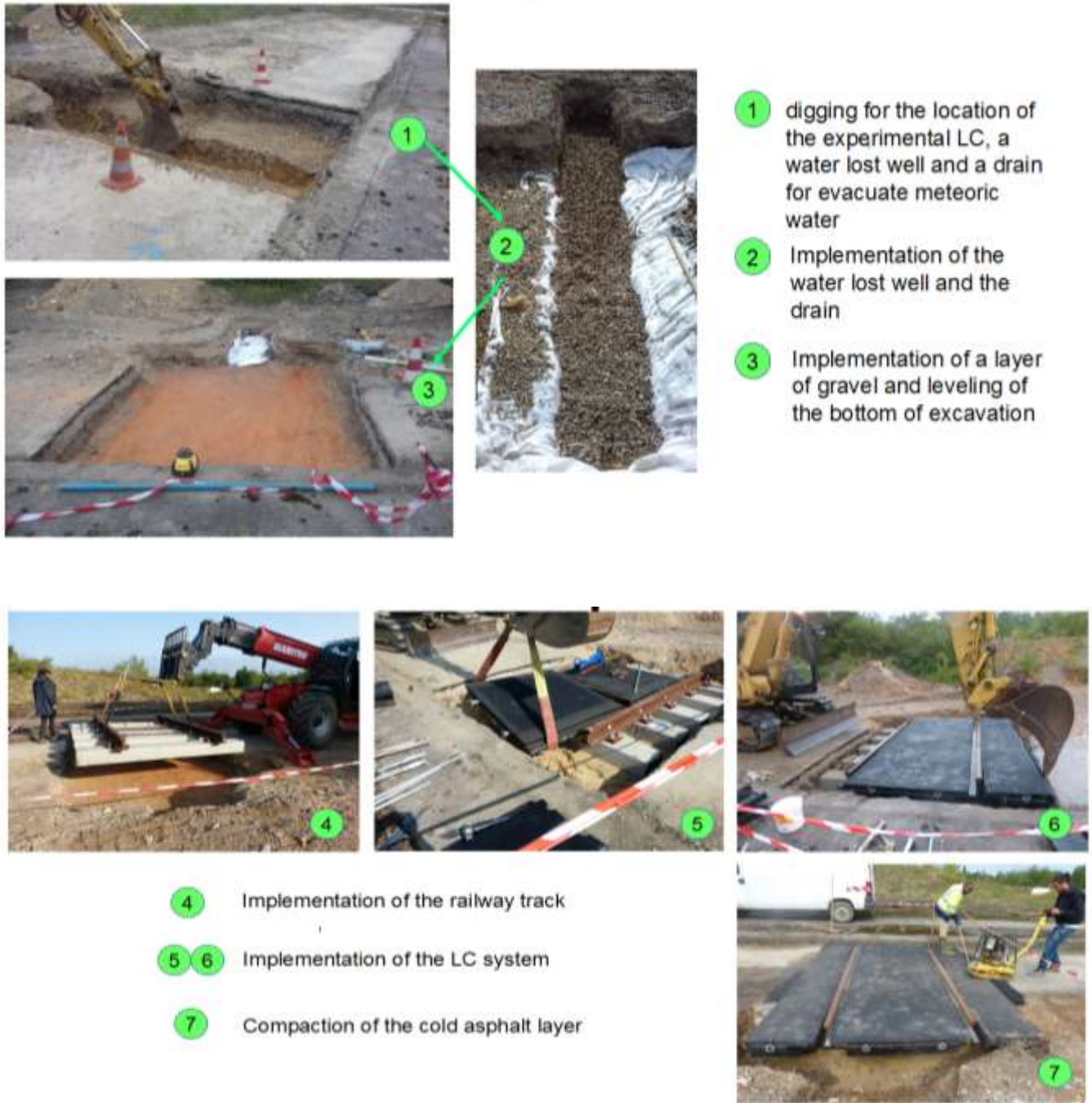
Figure 12. Experimental level crossing implementation (Cerema test site)
