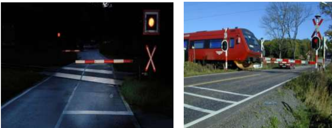
Figure 48: Level crossing with light signal and half-boom.
